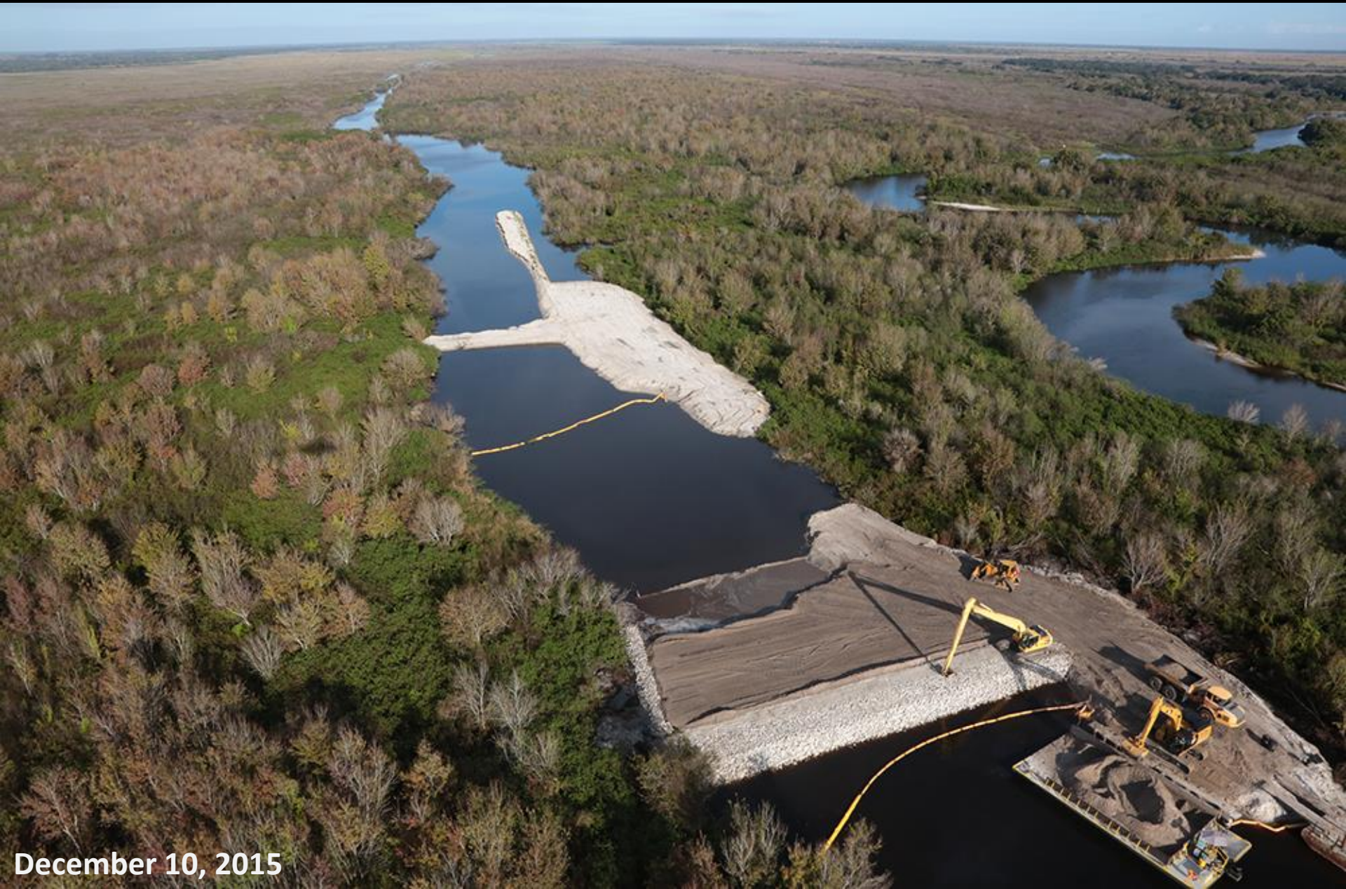
Looking north (upstream) from the southern end of the MacArthur Ditch backfill project where a rock plug was installed. Backfilling of the ditch has been resumed.
