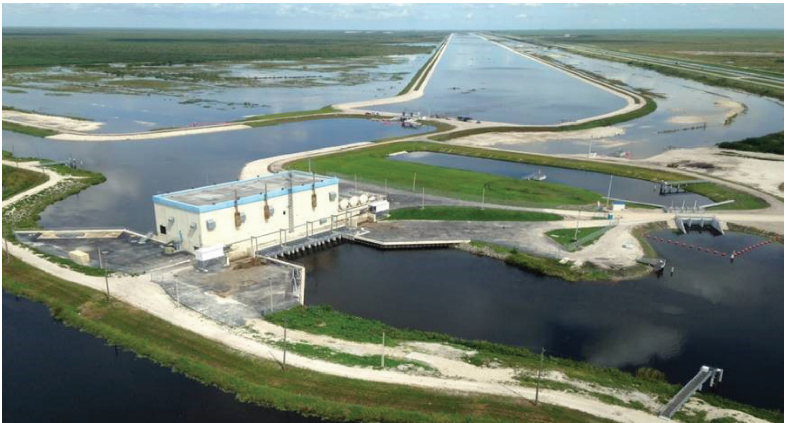
Optimizing system performance: Completed ahead of schedule in November 2015, the A-1 Flow Equalization Basin in Palm Beach County, which is part of Florida’s Restoration Strategies Plan for clean water for the Everglades, assists in optimizing the performance of two nearby stormwater treatment areas in removing phosphorus. It can hold up to 60,000 acre-feet of water up to 4 feet deep, and then delivers water in a controlled manner to the treatment areas. It is surrounded by 21 miles of levees and has 15 associated water control structures.
