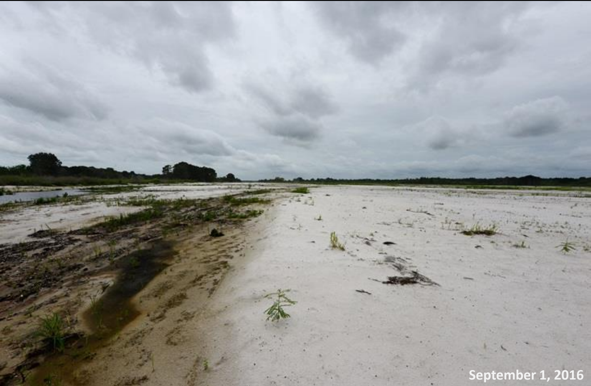
Lower section of Reach 3 backfill. This section of backfill was completed a couple months ago, and the backfill is beginning to vegetate.
