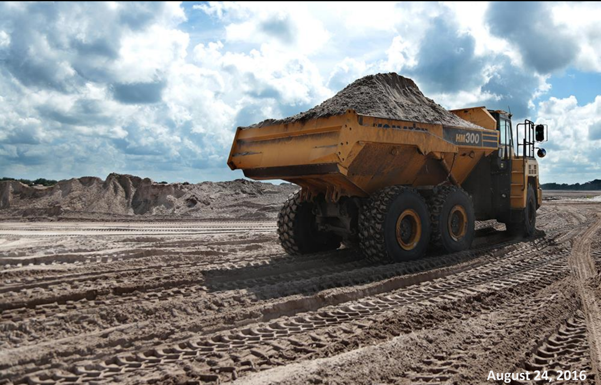
The final loads of spoil for Reach 3 C-38 backfill are hauled across the floodplain.
