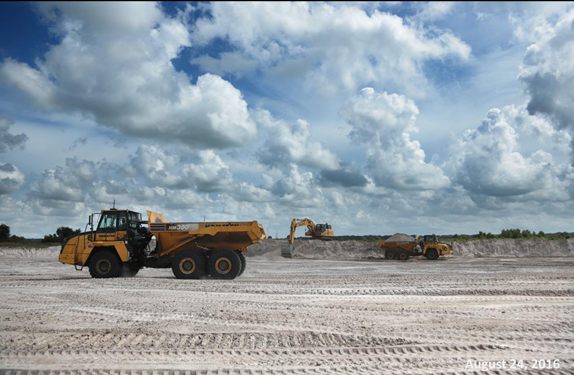
Degrading of the spoil pile in the Reach 3 construction area.
