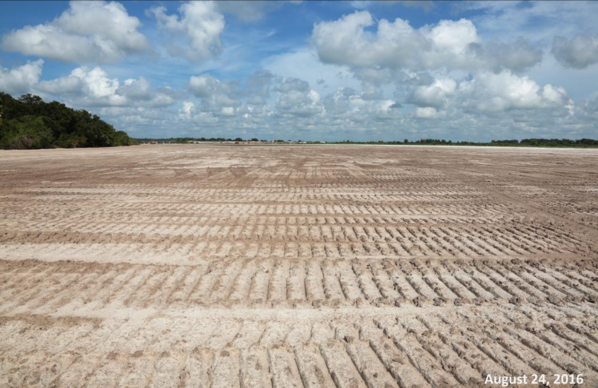
The C-38 canal has been backfilled, leveled and graded in the Reach 3 construction area, northern section just below HW98.
