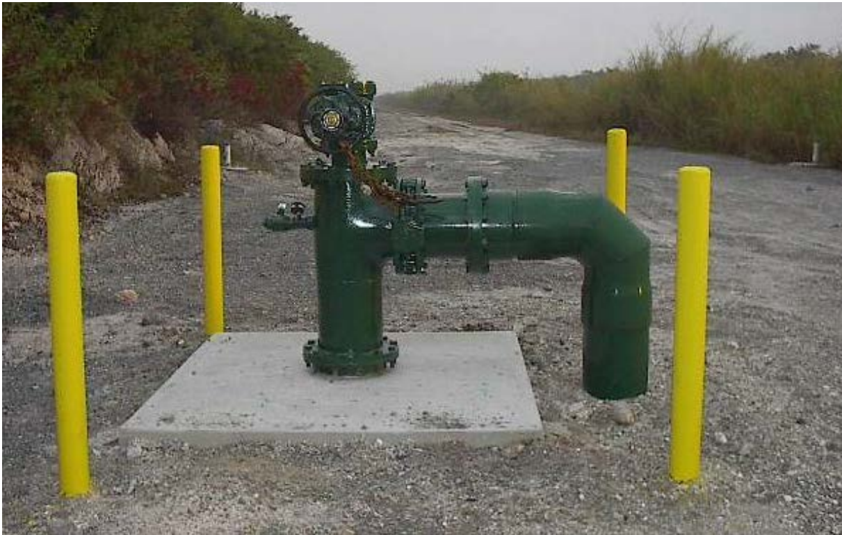
Figure 4. Completed Wellhead – Test/Monitor Well (MF-37)
