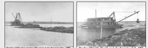
Construction of the Lake Surprise causeway circa 1905-1907. Photos from J. Wilkinson, keyshistory.org
