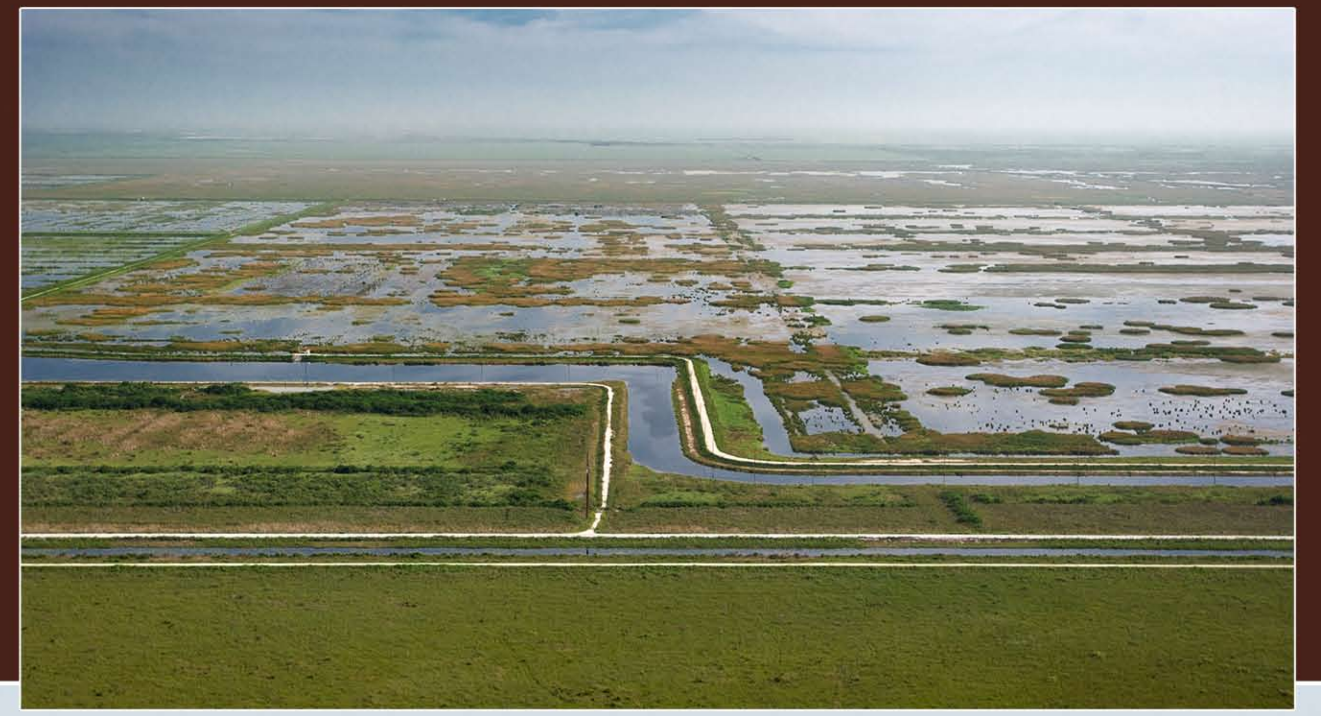
Stormwater Treatment Area 3/4 in Palm Beach County
