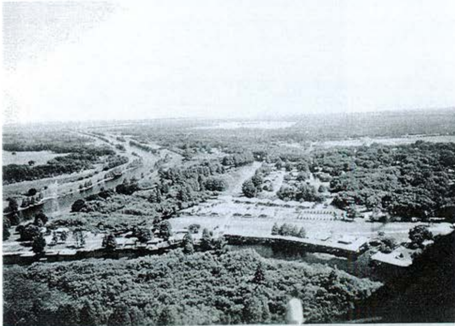
WEST SIDE OF C-37 LOOKING SOUTHEAST RAY LEIS PROPERTY ( KISSIMMEE RIVER PARK) IN FOREGROUND
