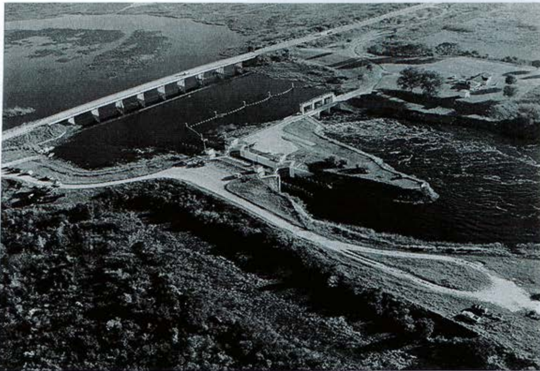
PHOTO A-7 S-65, Lock Structure and Operator's Residence (Looking from southwest towards S.R. 60 Bridge)
