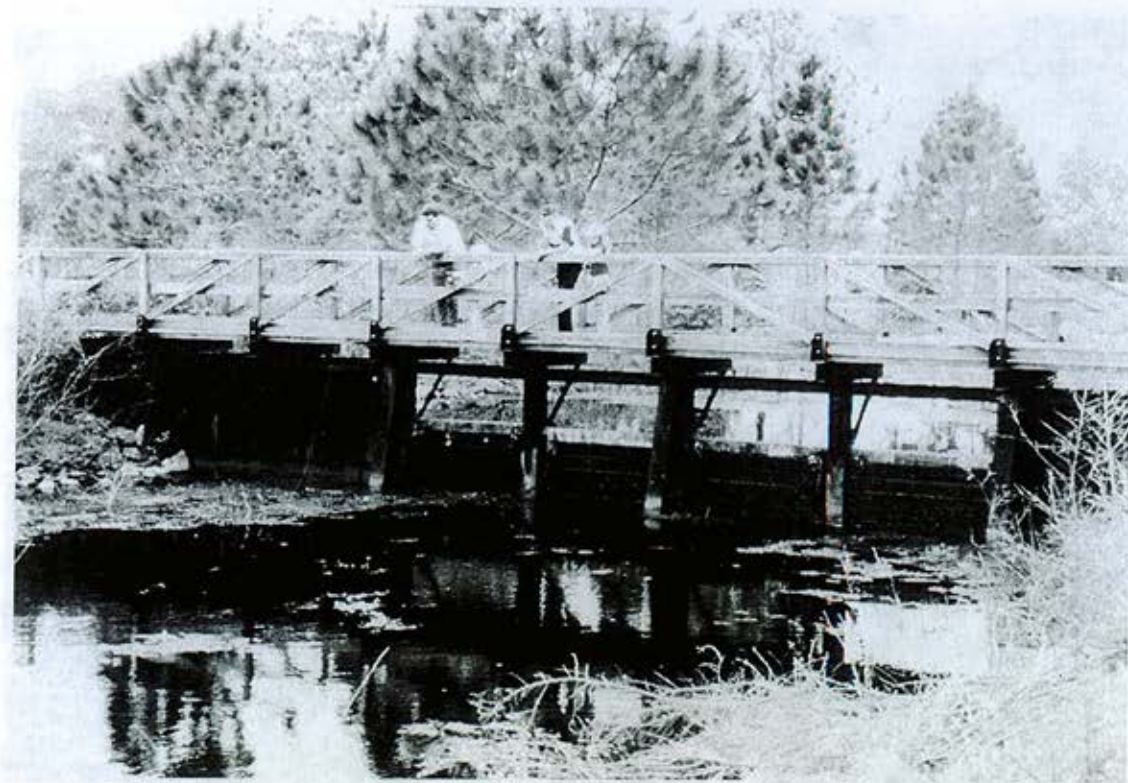
PHOTO A-10 Lake Rosalie Control Structure, G-103 (Downstream Side)
