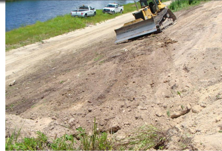
C-14 Levee Reshaping
