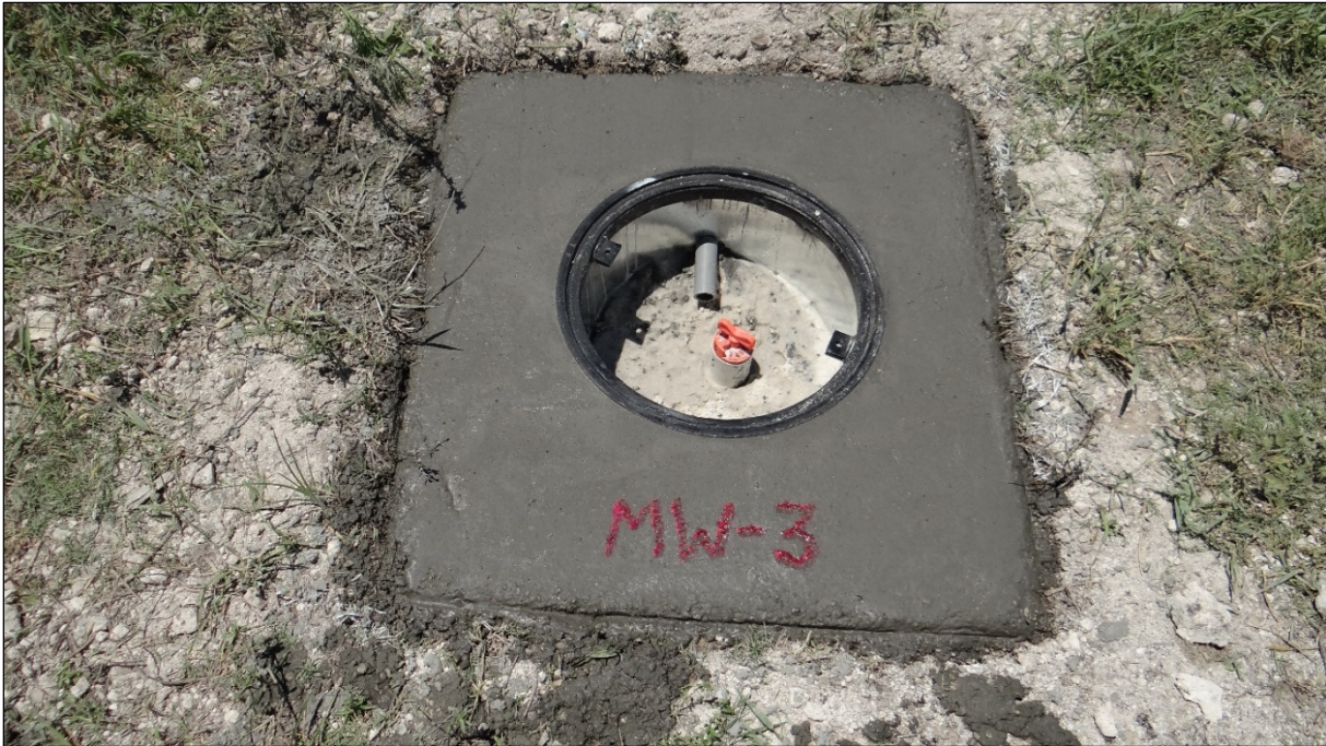
Figure 5. Completed monitor well.
