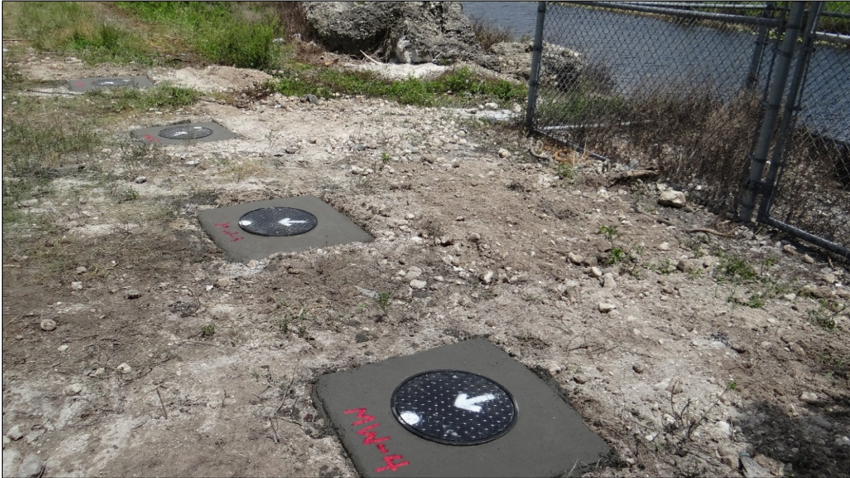
Figure 4. Completed wellheads (photo looking east-southeast).
