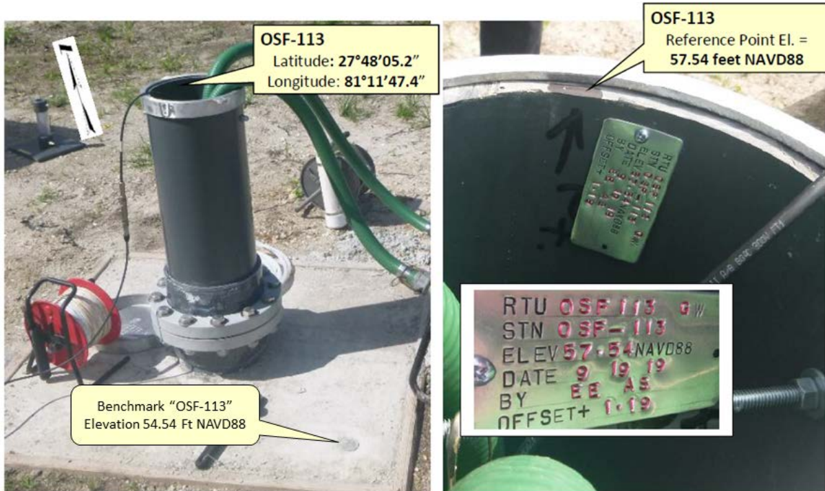
Figure 3. Completed OSF-113 wellhead, showing surveyed horizontal and vertical positions and measuring point (reference) location for depth-to-water measurements.
