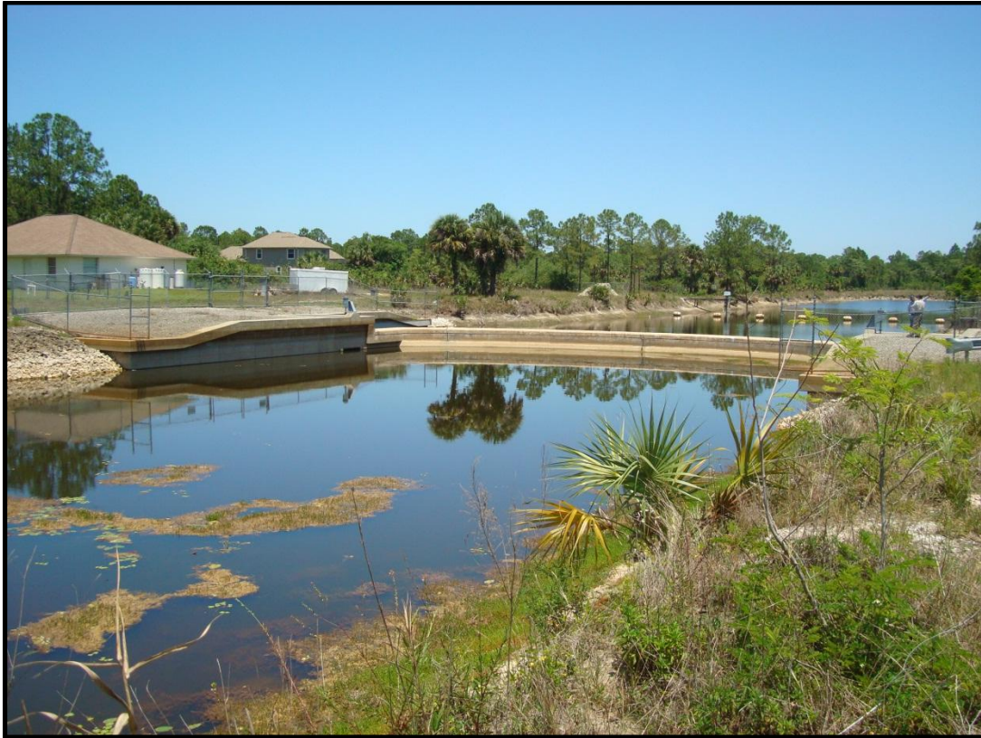
Photo 2 - GG4 Downstream View
