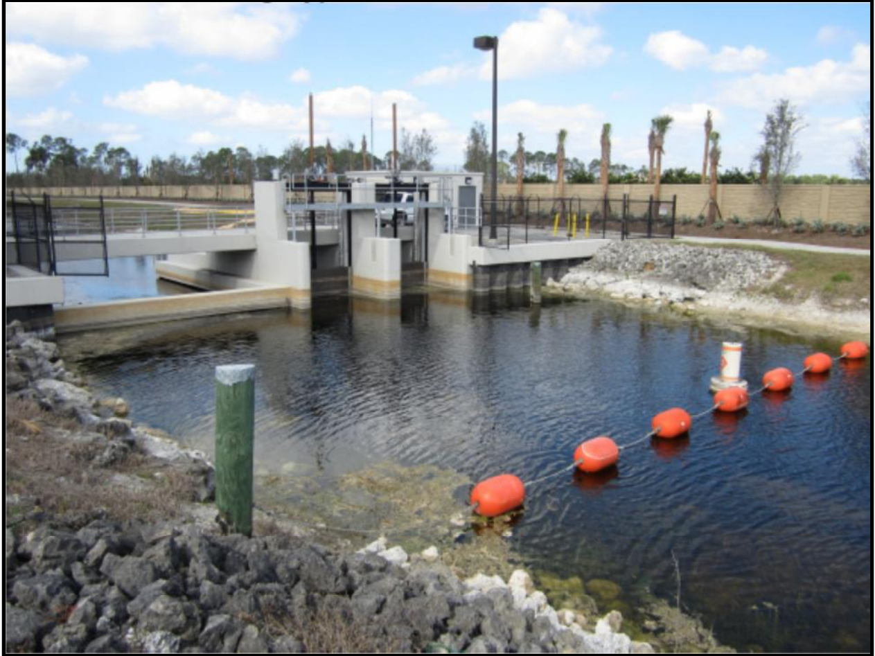
Photo 4 – Typical COCO Structures (COCO3 Upstream View)
