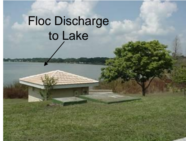
Underground Alum Storage Tank
