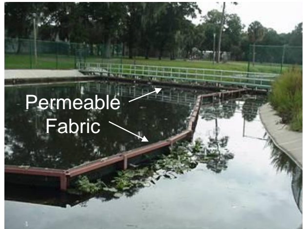
Figure 2-7. Overview of the Gore Street Alum Stormwater Treatment System.
