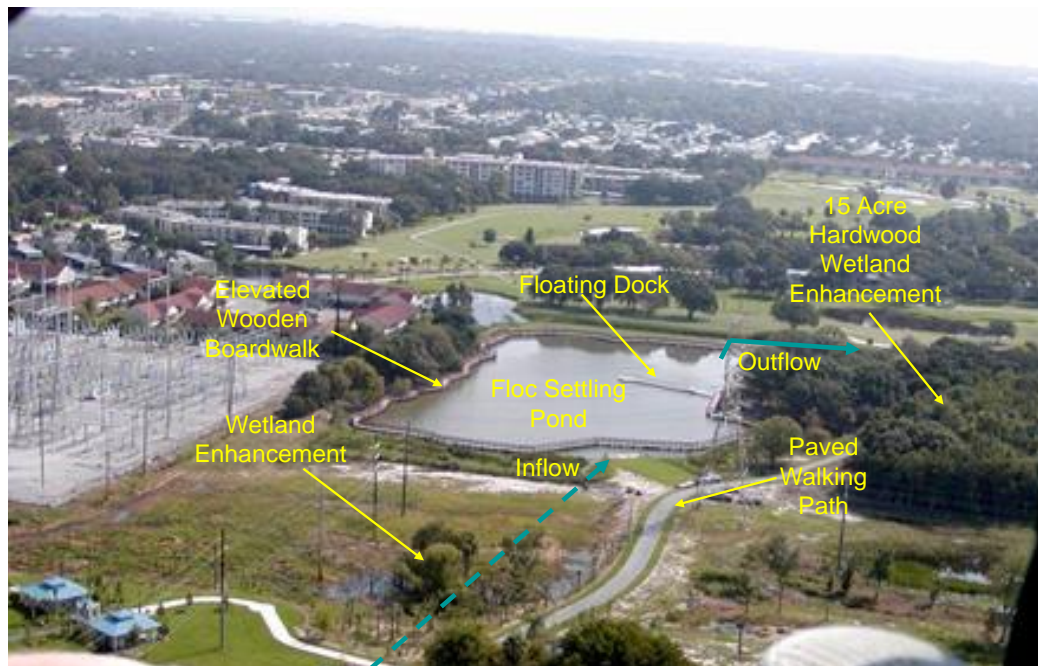
Figure 2-8. Overview of the Largo Regional Alum Treatment Facility.
