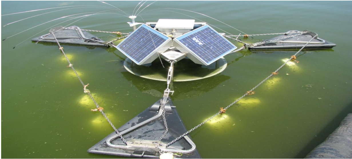
Figure 3-5 SolarBee system showing Floc Logs attach
