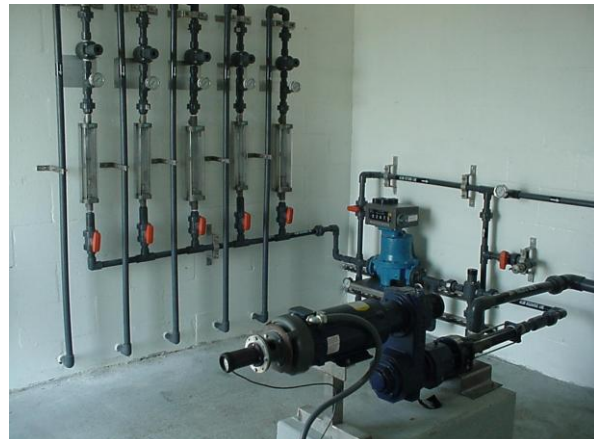
Figure 2-5. Overview of the Lake Howard Alum Stormwater Treatment System.
