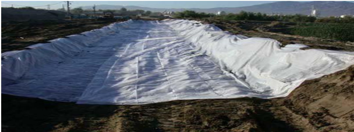
Figure 3-2 Treatment ditch lining to prevent soil contamination
