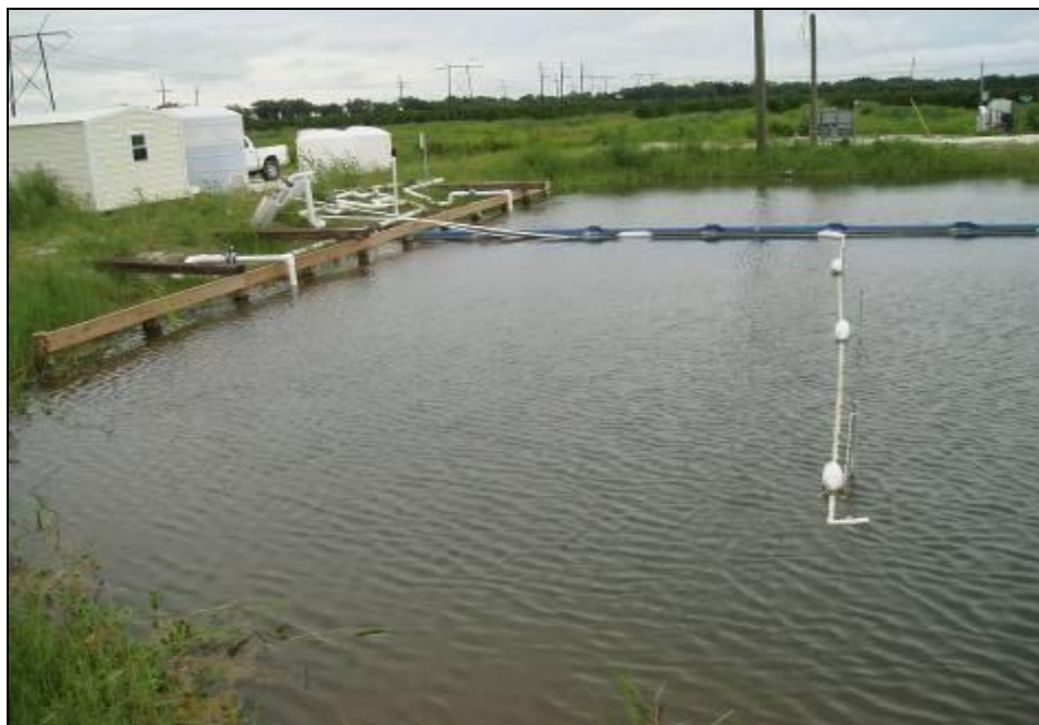
Figure 5-8. Floc recirculation infrastructure on the southern (B) HWTT flow path.
