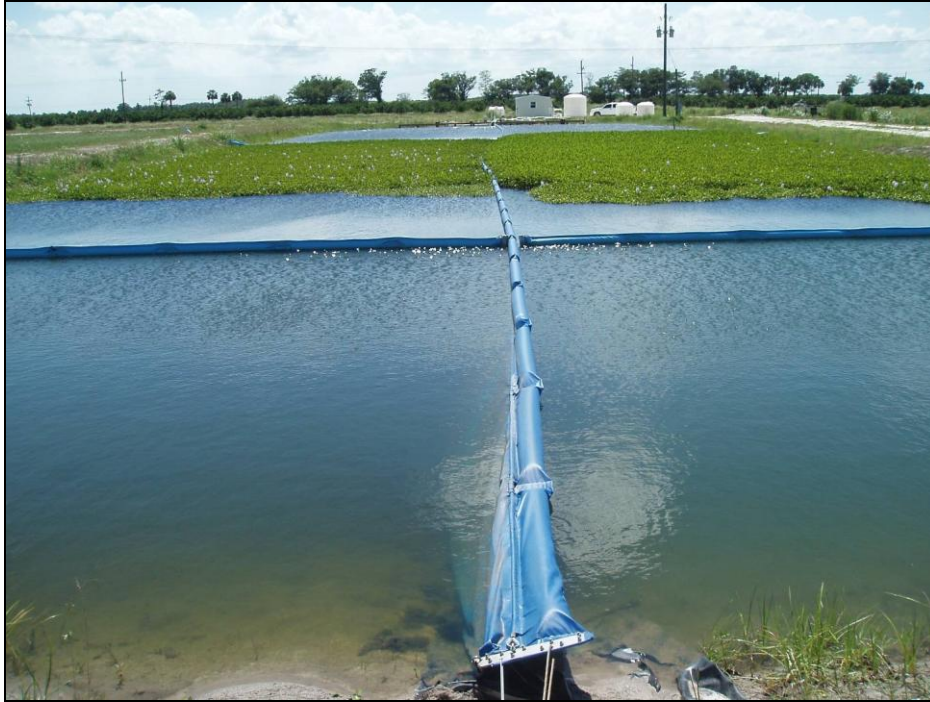
Figure 5-6. The outflow region of the Ideal Grove HWTT, with the northern (A) flow path on the right, and the southern (B) flow path on the left. The northern flow path receives continuous amendment additions, while the southern flow path receives amendments only intermittently.
