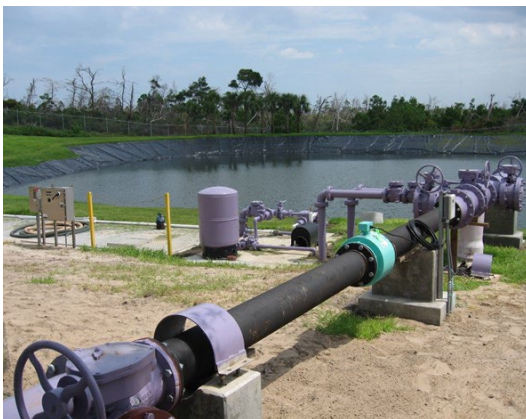
Reclaimed Storage Pond and Pump Station
