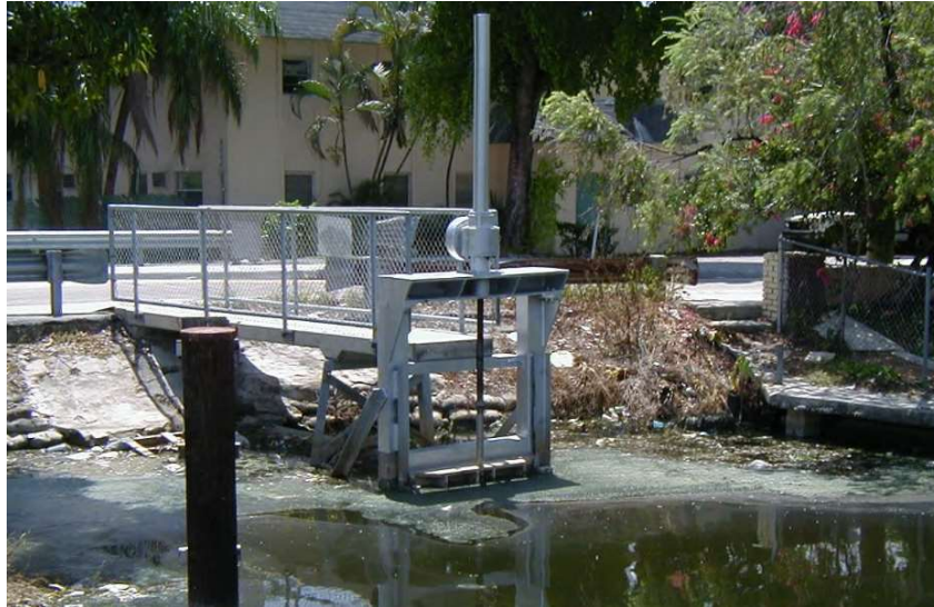
Figure 33: Current S-25A structure
