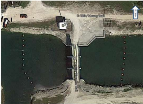
Figure 1 – Aerial image of the S20F Structure site
