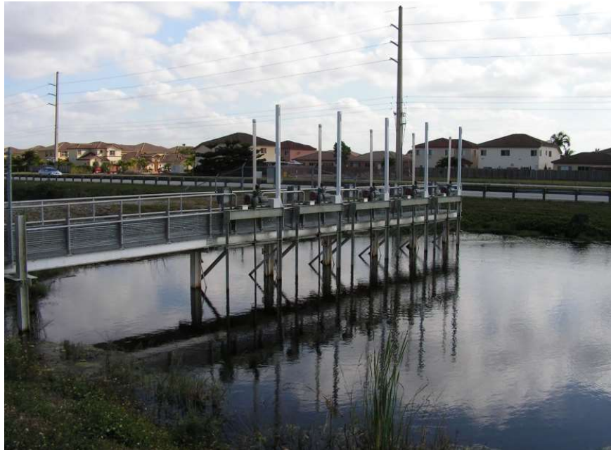
Figure 38: Current S-380 structure
