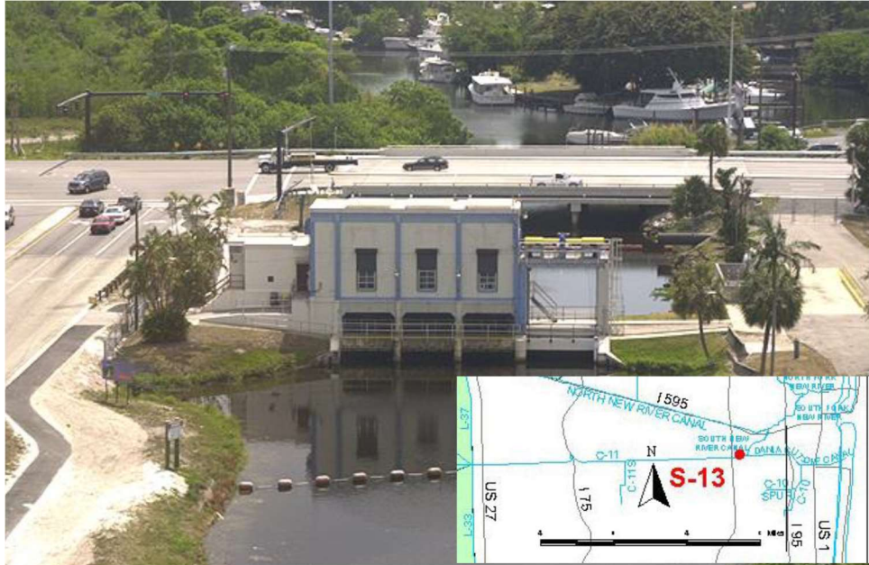
Figure 22: Structure S-13 – Upstream View (Photo by SFWMD)
