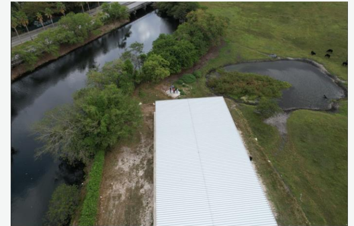
Site Reconnaissance Survey at W.H. Turner School NBS Site
