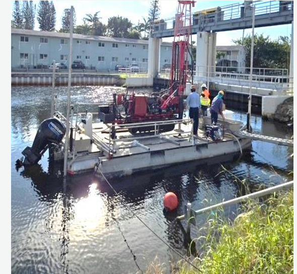
Geotechnical Investigation at S-27 Spillway
