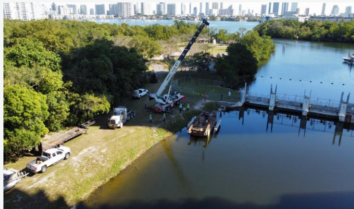
Geotechnical Investigation at S-29 Spillway
