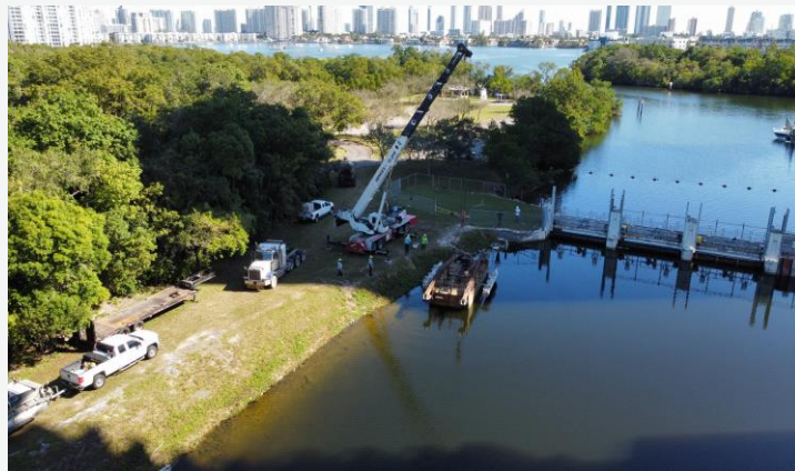
Geotechnical Investigation at S-29 Spillway
