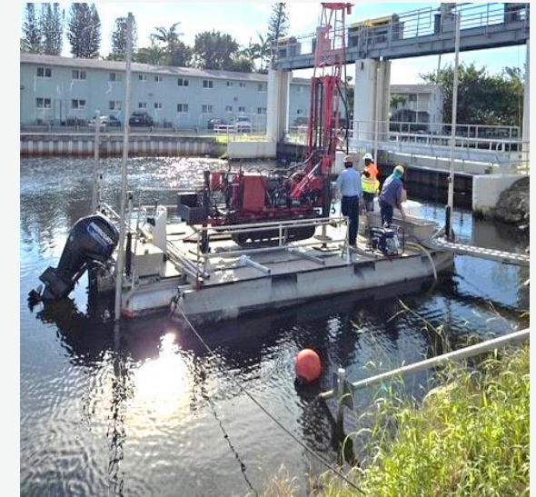
Geotechnical Investigation at S-27 Spillway
