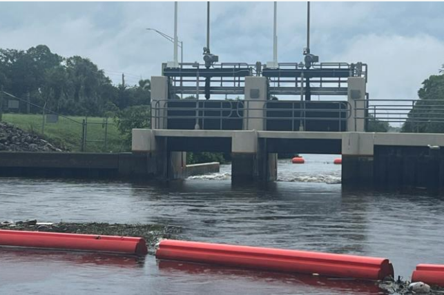
COCO1 (Coastal Structure)
