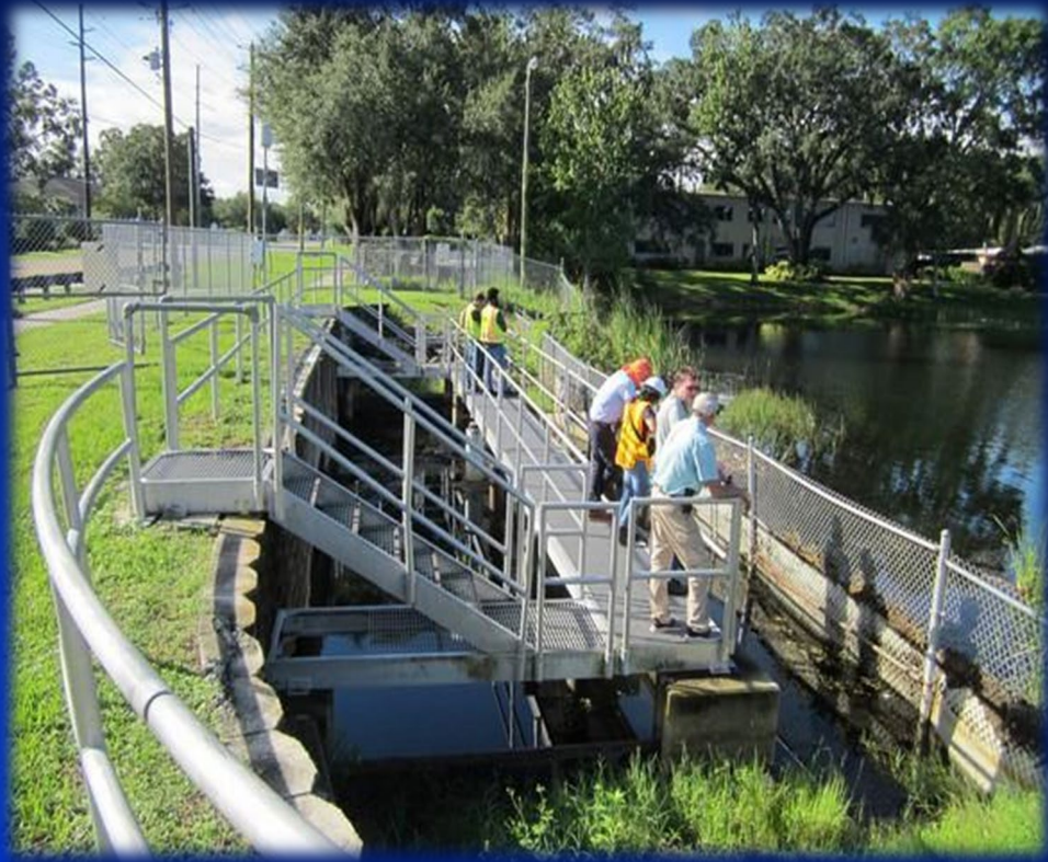
Daetwyler Control Structure
