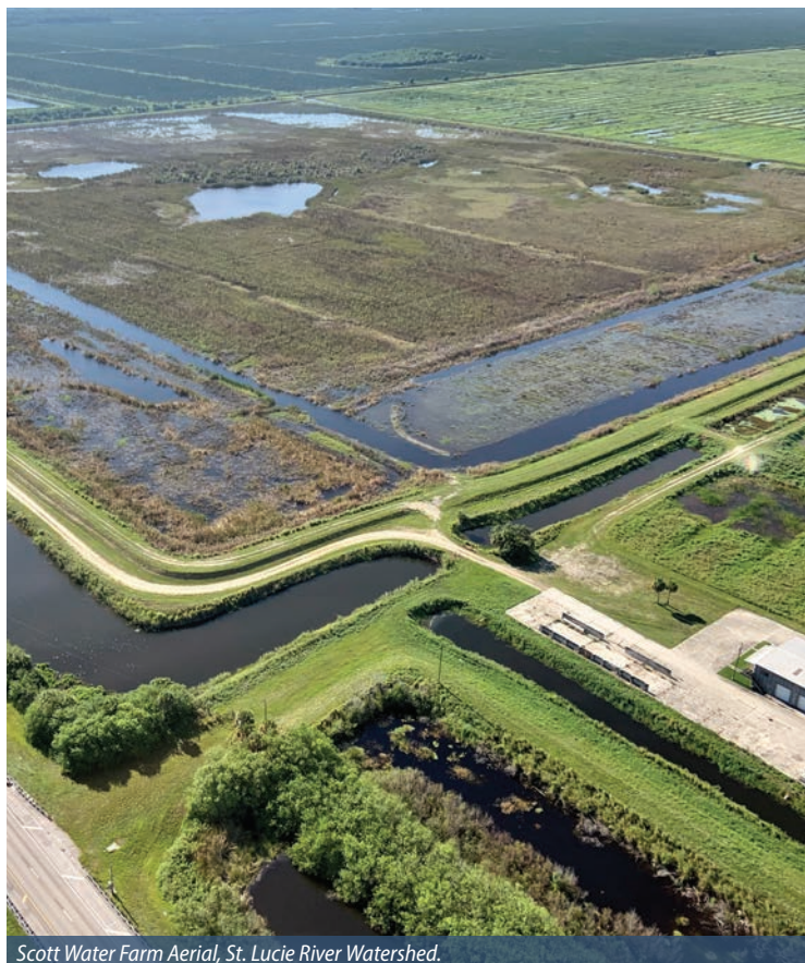
Scott Water Farm Aerial, St. Lucie River Watershed.
