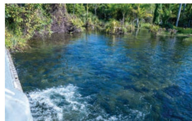
Downstream of Deering Estate Pump Station Spreader.
