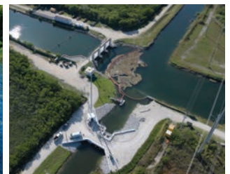
L-31 Flow Way Pump Station S-709.
