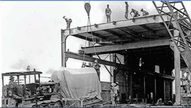
Moving One of the Engines into the S-5A Pump Station in 1954.
