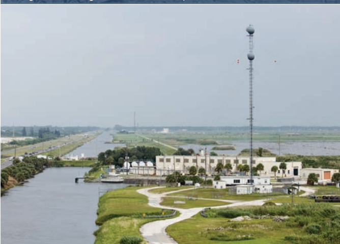
Modern Day S-5A Pump Station.
