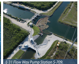
L-31 Flow Way Pump Station S-709.
