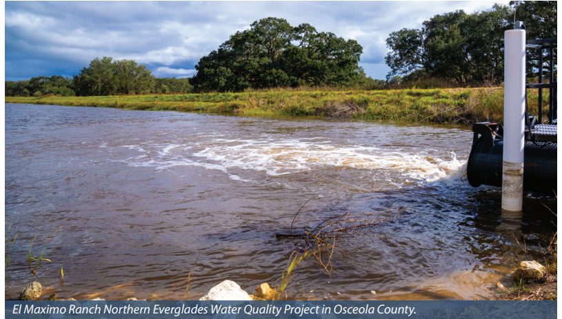
El Maximo Ranch Northern Everglades Water Quality Project in Osceola County.
