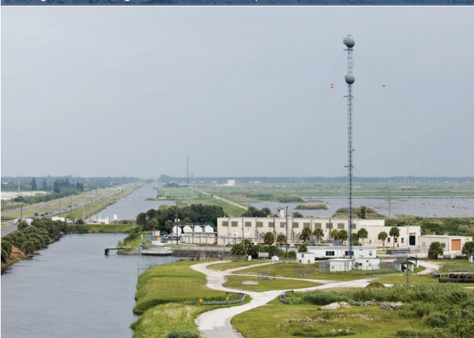
Modern Day S-5A Pump Station.
