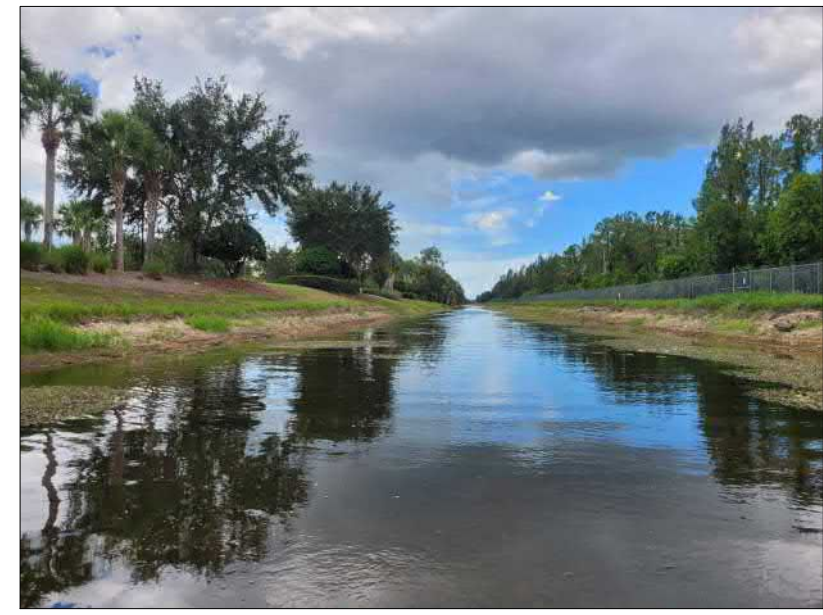
STATION 71+21 LOOKING SOUTH
