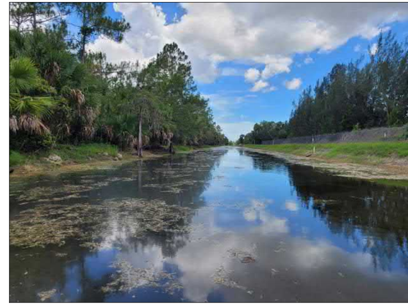
STATION 50+85 LOOKING SOUTH
