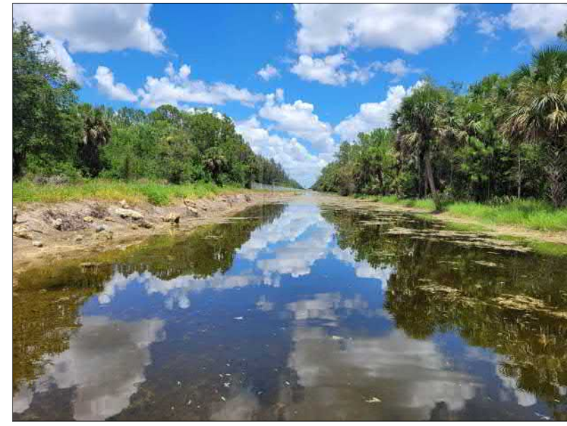
STATION 40+67 LOOKING NORTH
