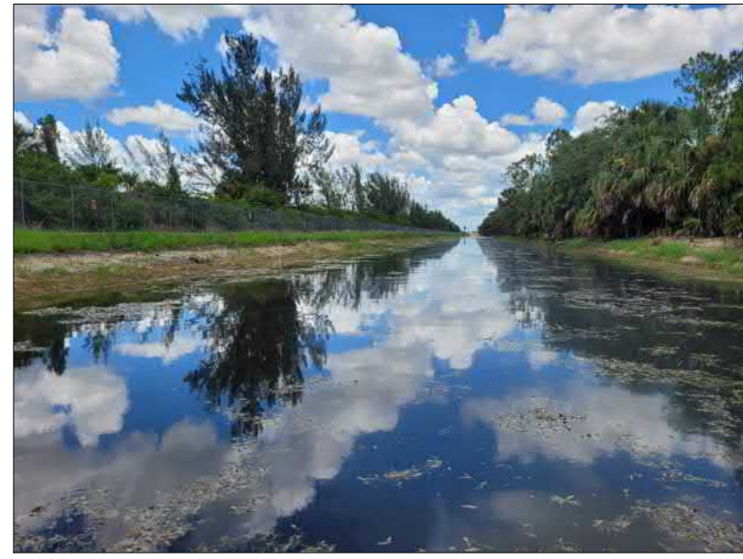
STATION 50+85 LOOKING NORTH
