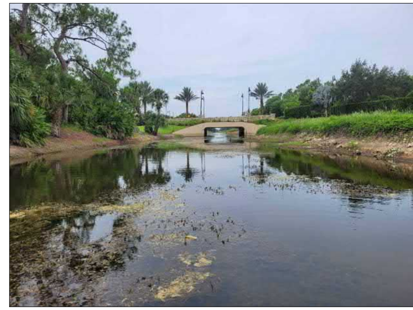
STATION 81+29 LOOKING SOUTH
