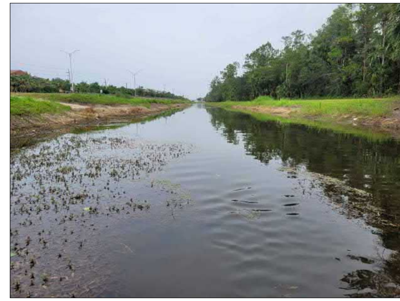
STATION 89+16 LOOKING NORTH
