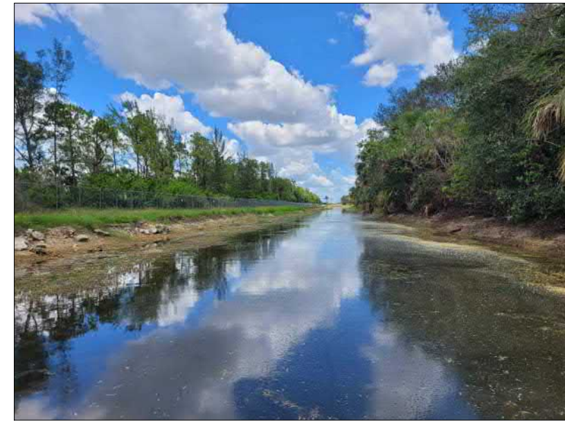
STATION 61+14 LOOKING NORTH
