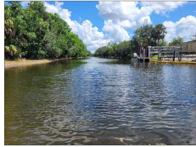
STATION 10+22 LOOKING NORTH
