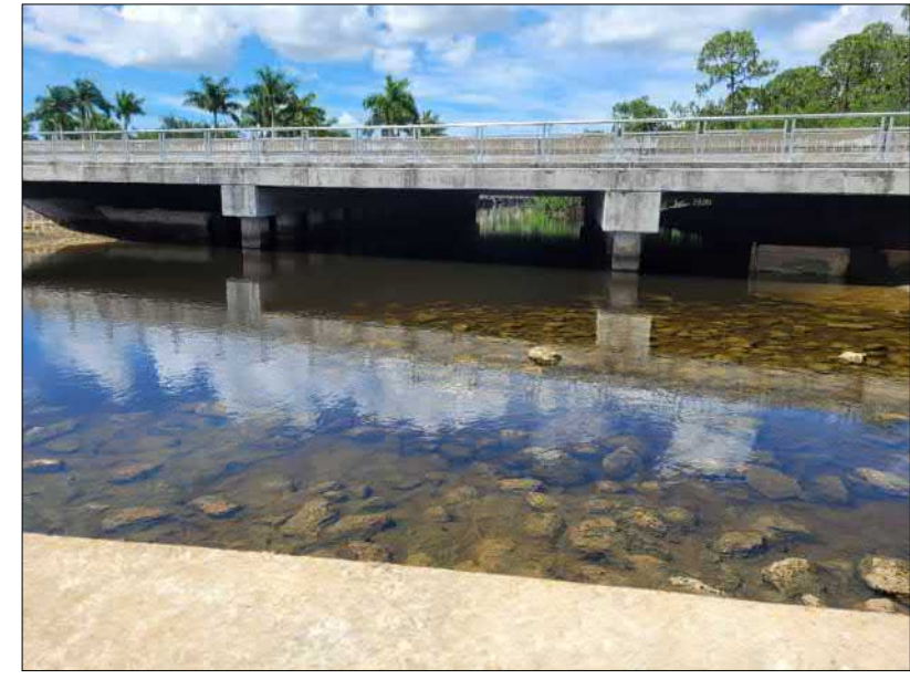
STATION 10+22 LOOKING SOUTH
