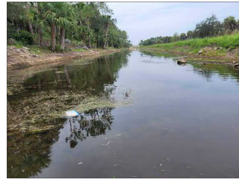
STATION 89+16 LOOKING SOUTH
