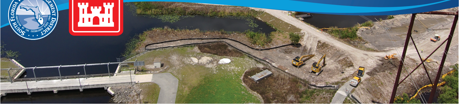
Construction at CEPP North.
