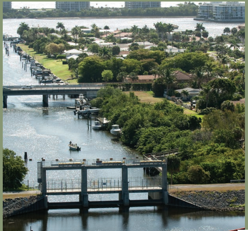
C-51 Gate Structure
