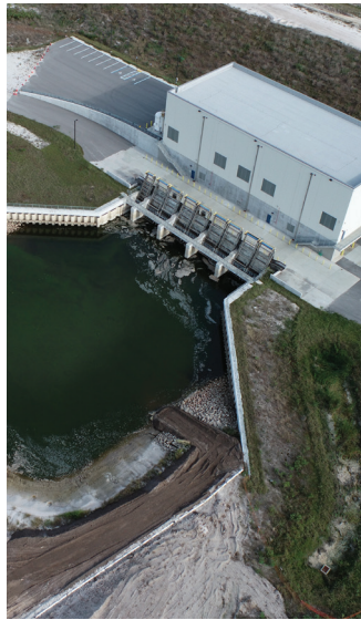
S-470 Pump Station at the Caloosahatchee (C-43) Reservoir.
