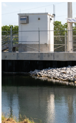
Pump Station S-709.
