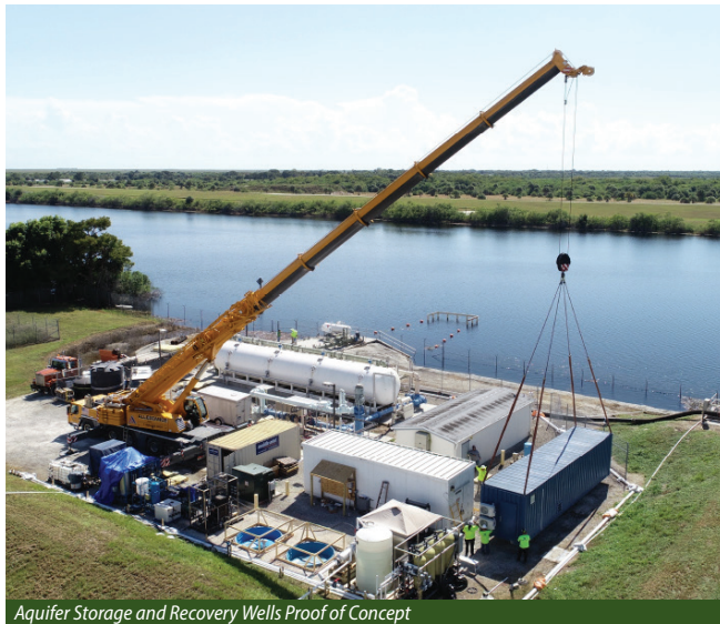
Aquifer Storage and Recovery Wells Proof of Concept
