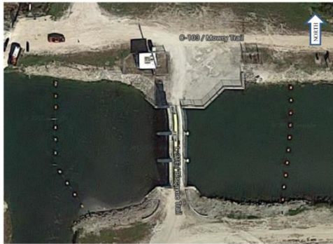
Figure 1 – Aerial Image of the S20F Structure site
