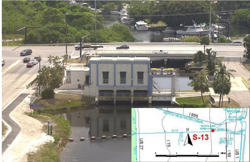
Figure 22: Structure S-13 – Upstream View (Photo by SFWMD)
