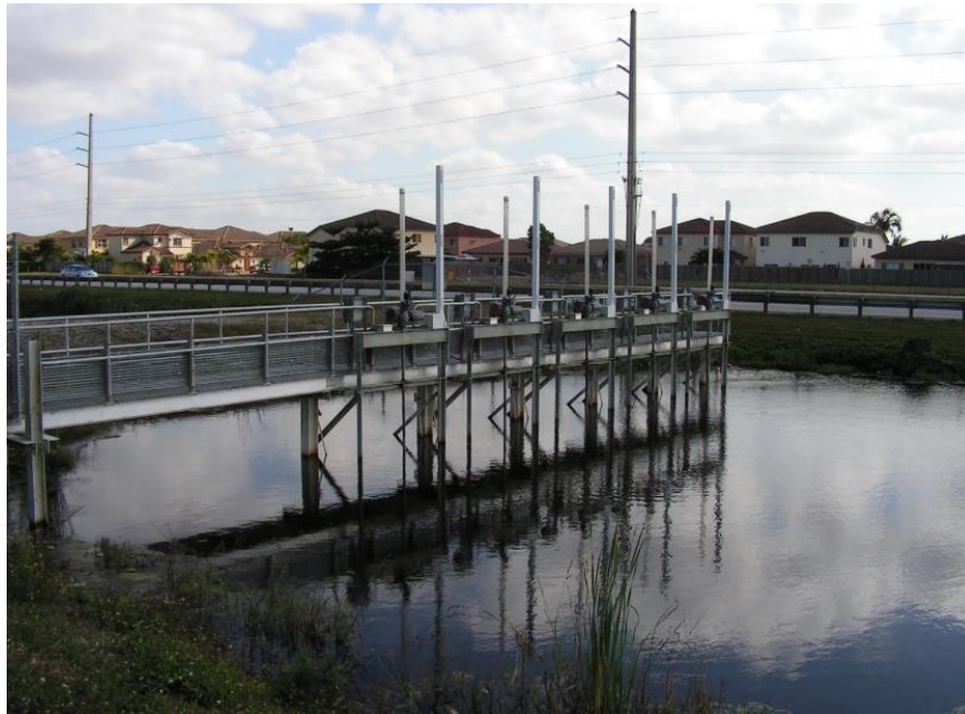
Figure 38: Current S-380 structure.
