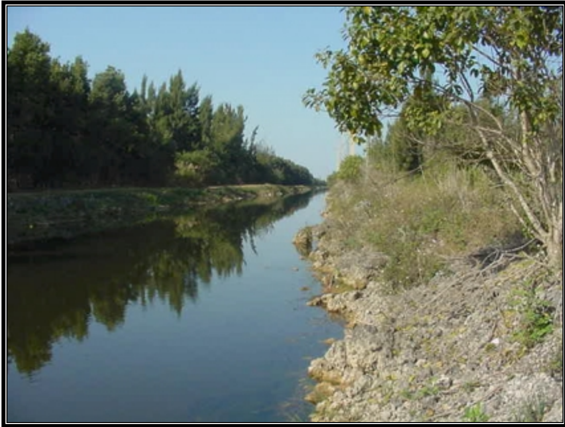
3) View of east-west trending canal located on the southern boundary of Study Area 5.
