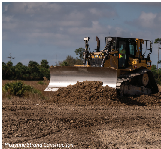
Picayune Strand Construction
