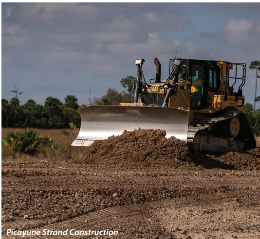
Picayune Strand Construction
