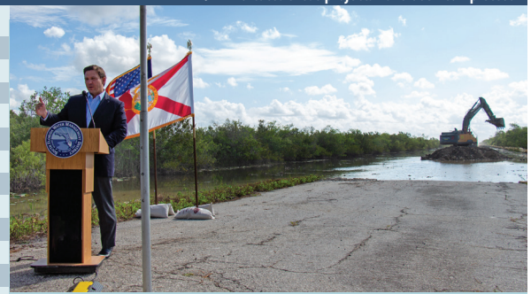
Gov. DeSantis at the Old Tamiami Trail Roadbed Removal Groundbreaking
