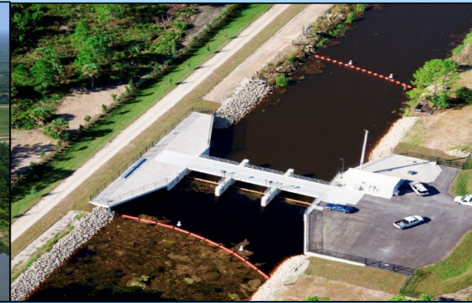
Golden Gate Structure 3 (GG3)
