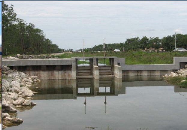
Henderson Creek Structure 2
