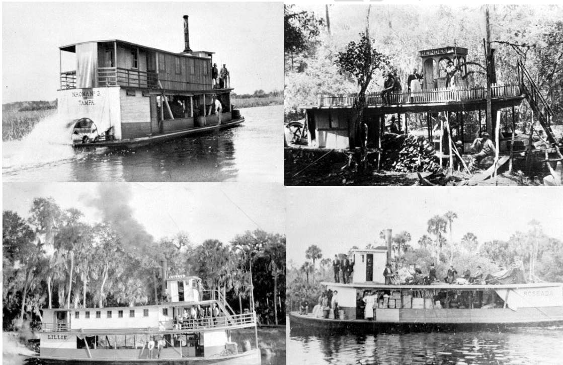
The 50-foot sternwheel steamers of the Kissimmee River system, clockwise from upper left: the Naoma, the Talullah, the Roseada, and the Lillie.
