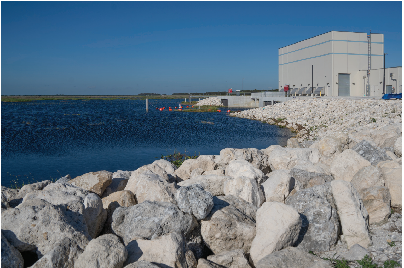
C-139 Flow Equalization Basin in Hendry County
