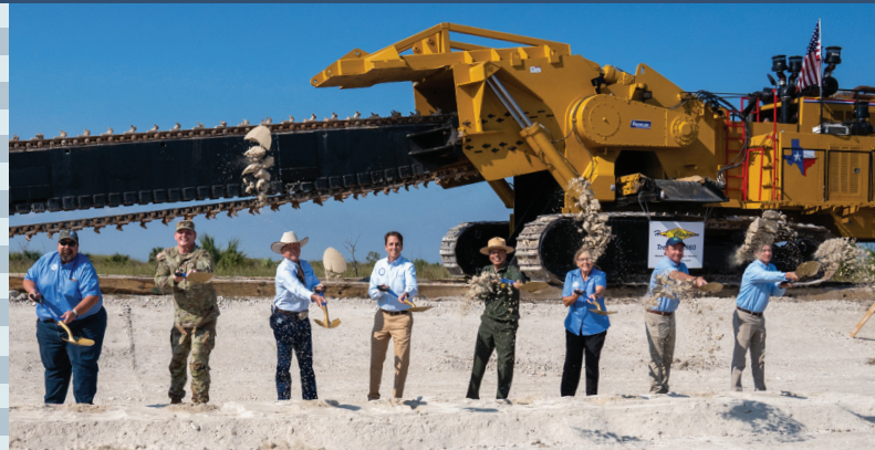
CEPP New Water Seepage Containment Wall Groundbreaking Ceremony
