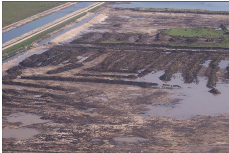
Figure 2. Photo of substrate preparation during PSTA cell construction. Organic soils were scraped from limerock, then removed or formed into berms that extend perpendicular to the dominant (north-to-south) flow direction.
