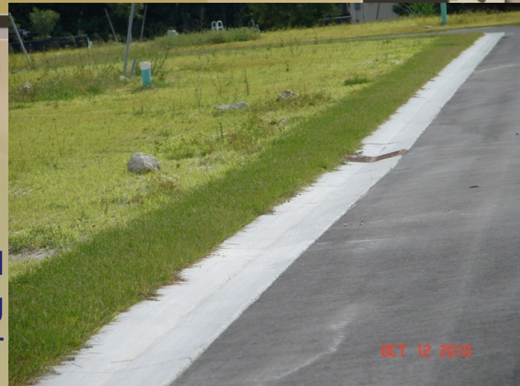
Hydroseeded and sod along curb gutter
