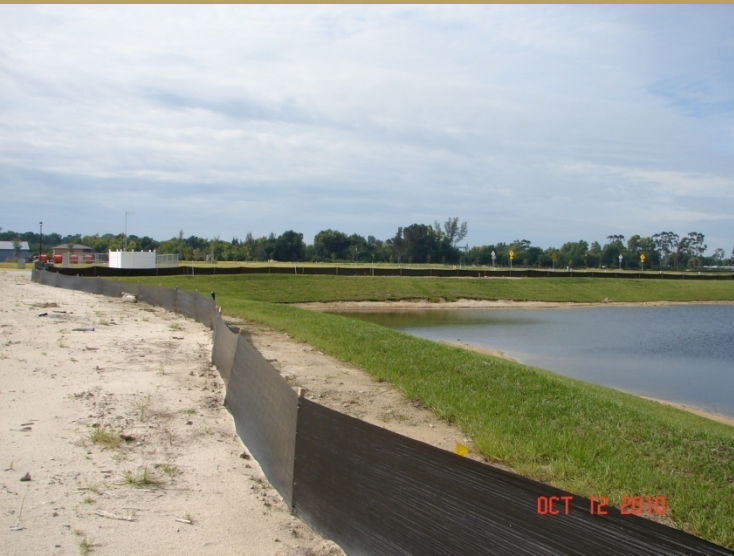
Silt fence and temporary diversion berm
