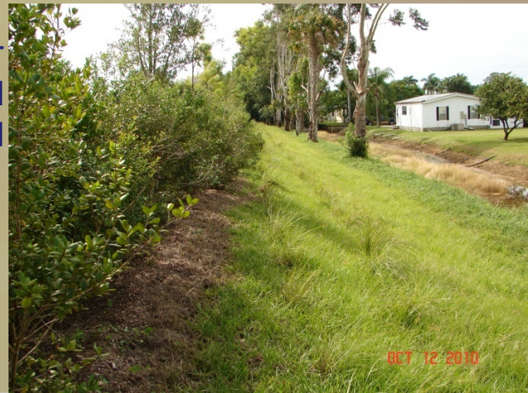
Perimeter berm stabilized and sodded
