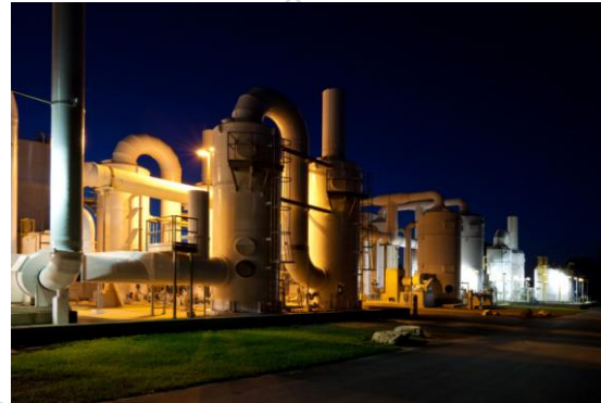
Collier County Water-Sewer District South County Regional Water Plant
