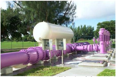
(Click on picture for larger version.) The color purple is used to identify pumps, tanks and pipes carrying reclaimed water for reuse.
