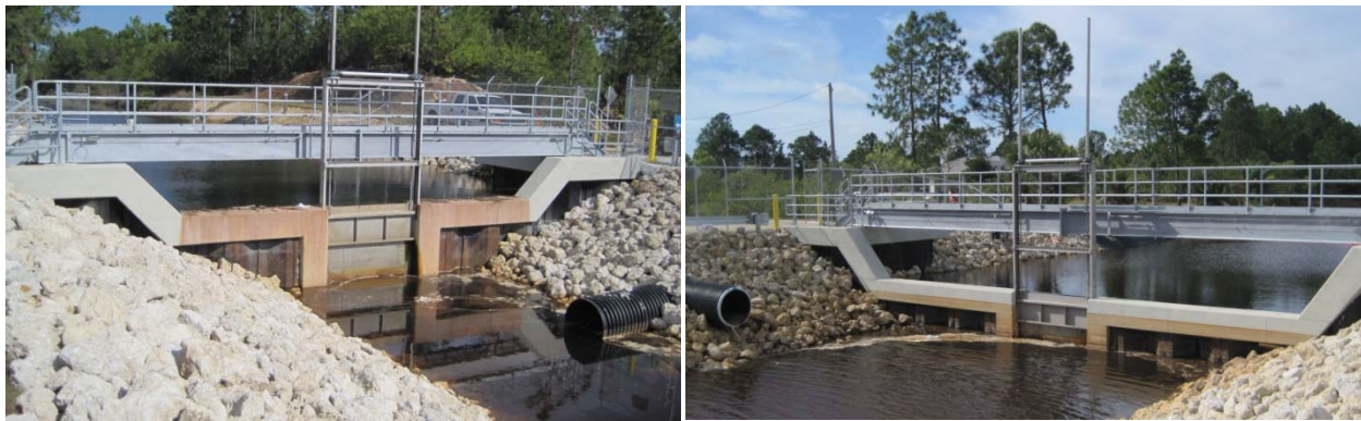
Golden Gate Main Canal Weir #6 (left), #7 (right). (Click on the pictures for larger versions.)
