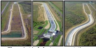
The project includes two pump stations, 10 plugs/water control structures and impoundments that can hold up to 1,200 acrefeet of water following rainfall events.
