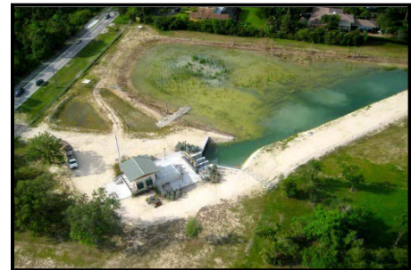
Aerial view of the constructed pump station and created wetlands at the Deering Estate Flow-way.
