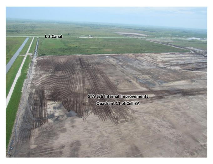
**STA-5/6 Internal Improvements:** Bulldozer tracks to spread material and achieve design grade elevation. View over Cell 3A facing west.
